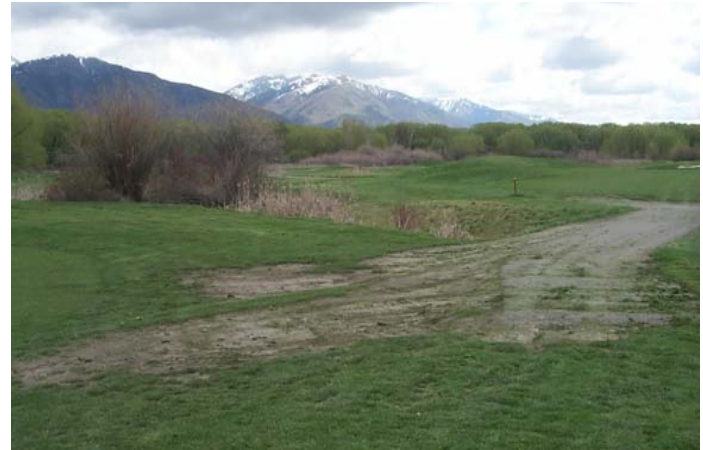
Needed Cart Path Repair #6 Fairway
