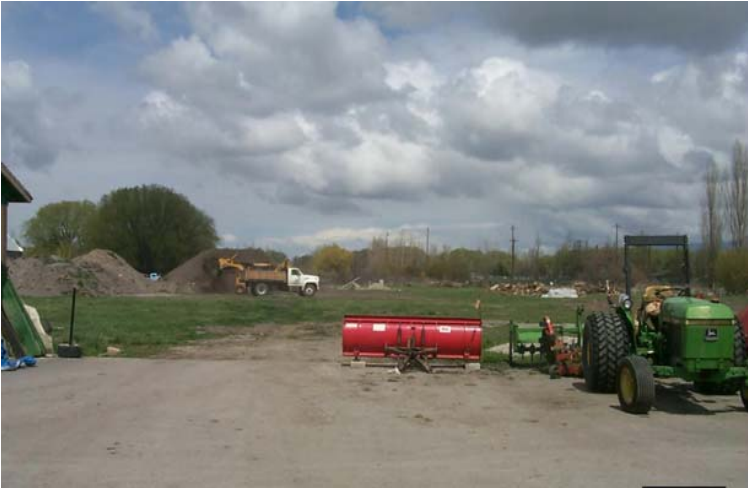
Maintenance Shop Improvements
