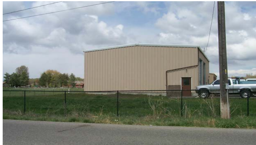
Maintenance Shop Entry Improvements
