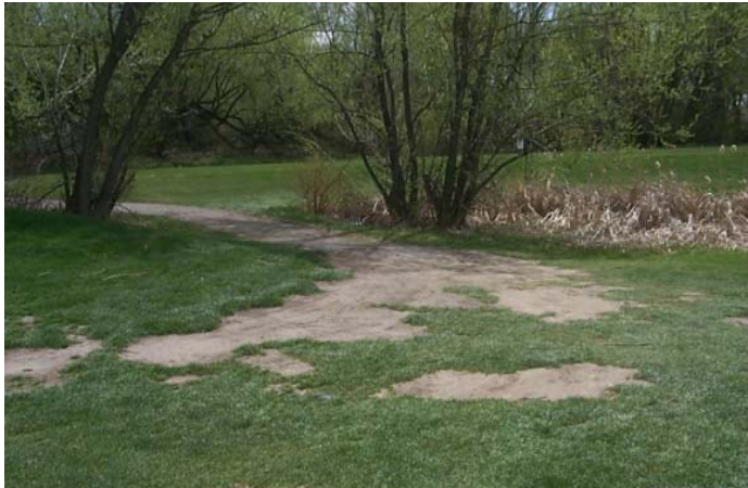
Needed Cart Path Repair #3 Green
